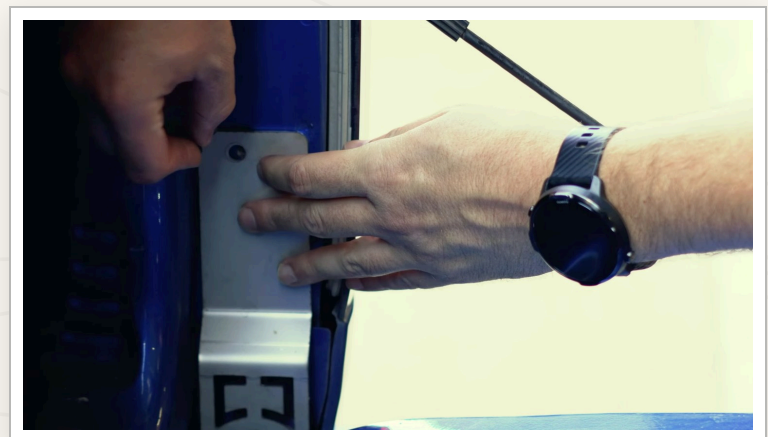
PLATE FLAT ON THE JAMB, BOLT STARTED BY HAND
