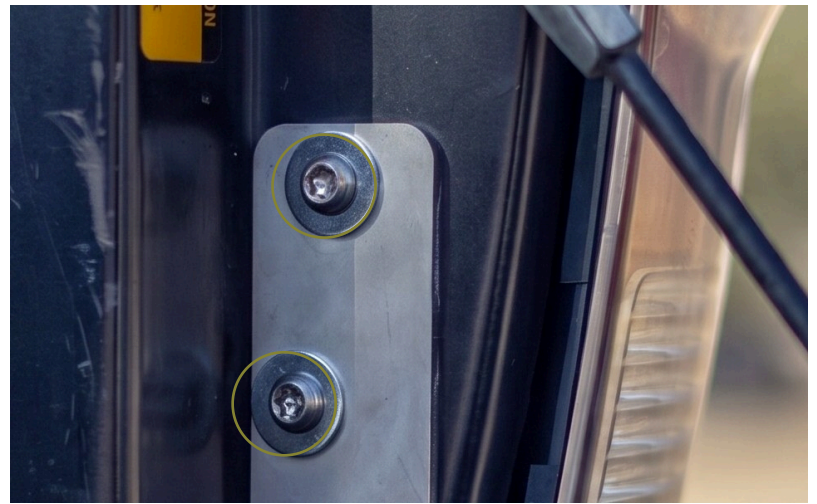
BOTH BOLTS SEATED, WASHER UNDER EACH HEAD, PLATE FLAT ON THE JAMB
